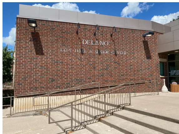
Delano, MN City Hall and Senior Center
